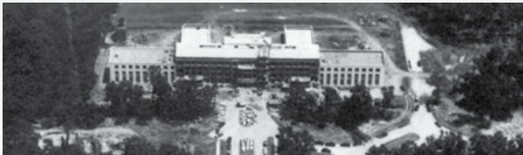
Baylor College of Medicine during construction in 1947.
