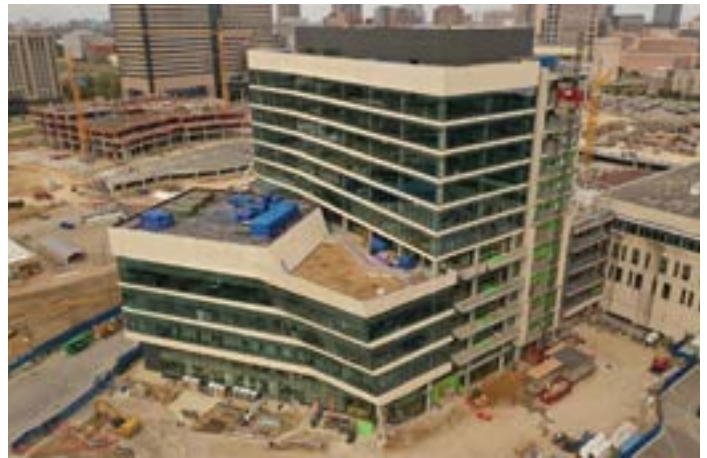
O'Quinn Medical Tower under construction.
